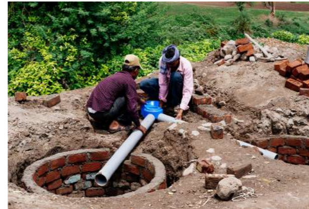
Installing SATO V-Trap
