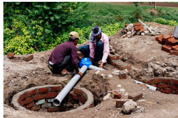
Installing SATO V-Trap toilet
