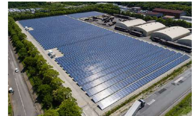
LIXIL Chita Plant in Japan
